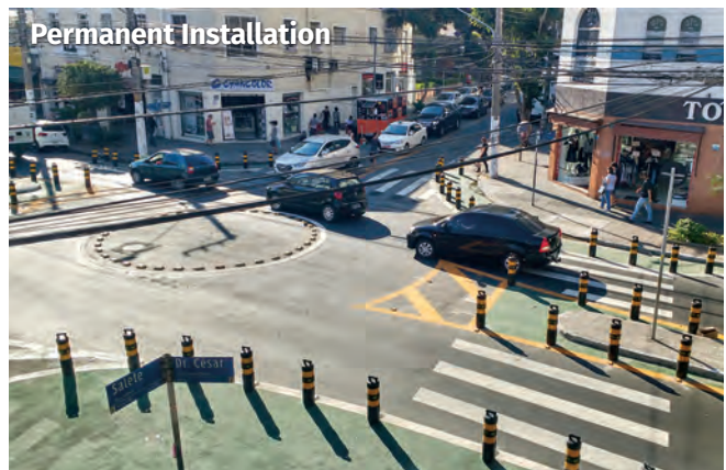
The Santana neighborhood of São Paulo was transformed with a pop-up installation, leading to a permanently improved intersection with traffic-calming measures and increased pedestrian safety. Photos: ITDP Brazil
